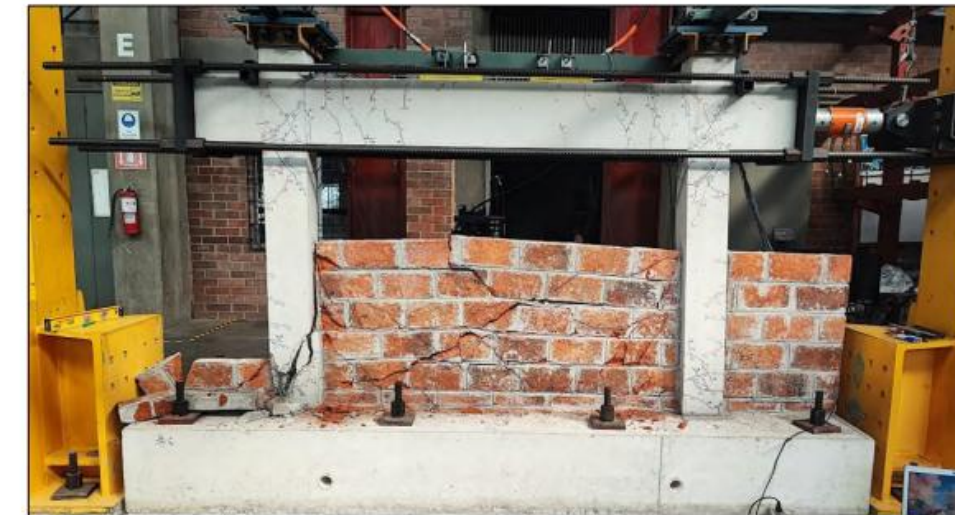
Fig. 3. 86 Final state of specimen SP-6 at a drift angle of 3.0%.
