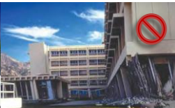
Original Olive View Hospital, Los Angeles, California.
