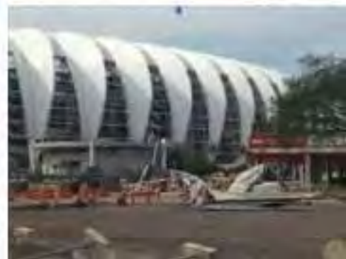
Full-scale damage to surroundings caused by downburst and no damage to stadium
